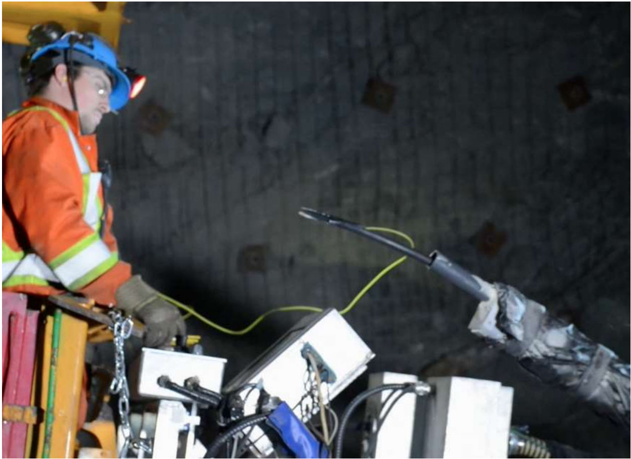
Figure 12 – Placing a Detonator into the Loading Hose.
