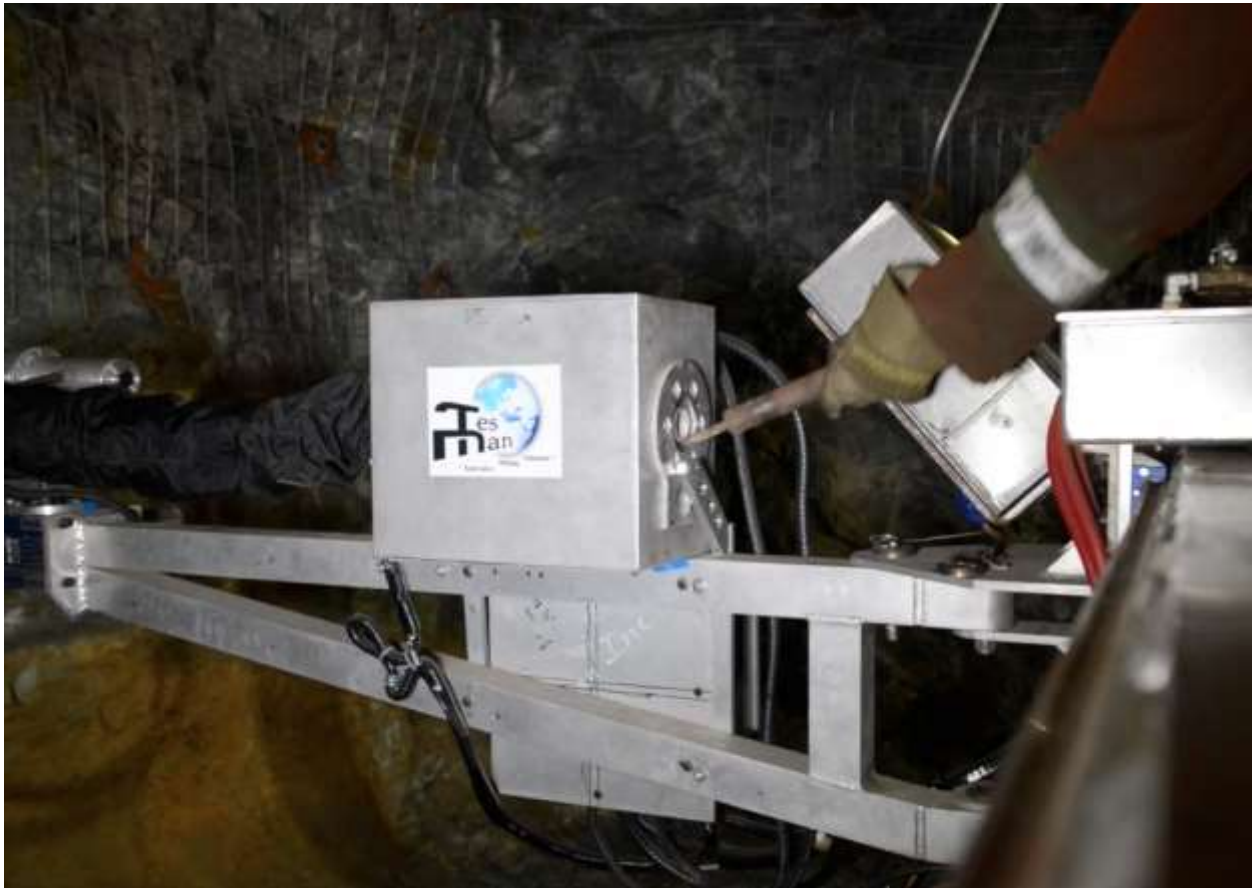
Figure 11 – Feeding the Impact Hammer into the Delivery Unit Ready for Use.
