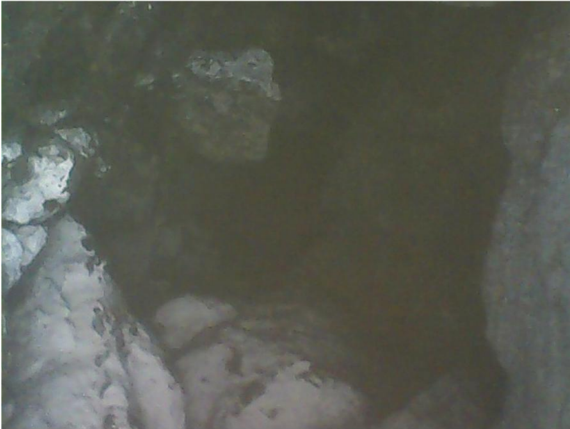
Figure 12: Typical Damage to Drill Hole Walls in Rock (Waste)
